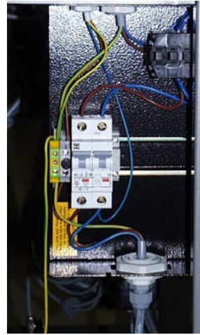
Fig 3-R-2 Fuse box 1 Phase models Cable diameter 9-12mm
