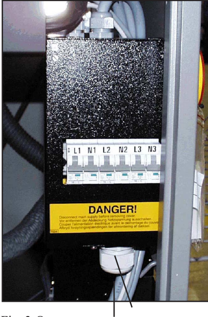
Fig. 3-Q Feed power cable through
